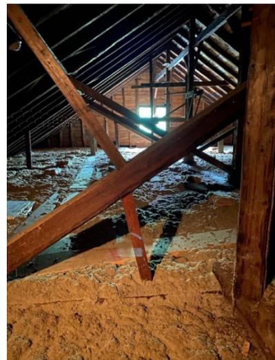
*Example of cellulose insulation in a timber-framed attic. Courtesy the Preservation Trust of Vermont.*
