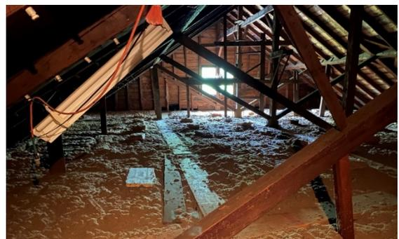
*This loose fill cellulose may be mess, but it can easily be removed to allow for repairs and preservation of historic features. Courtesy of the Preservation Trust of Vermont.*
