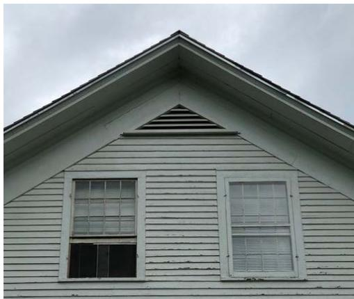
*Gable vents allow air to circulate under the roof, drying trapped moisture. Courtesy of the Preservation Trust of Vermont.*
