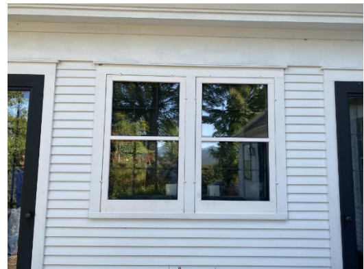
Wood storm windows fit tight around the window opening and can easily be removed. Courtesy of the Preservation Trust of Vermont.
