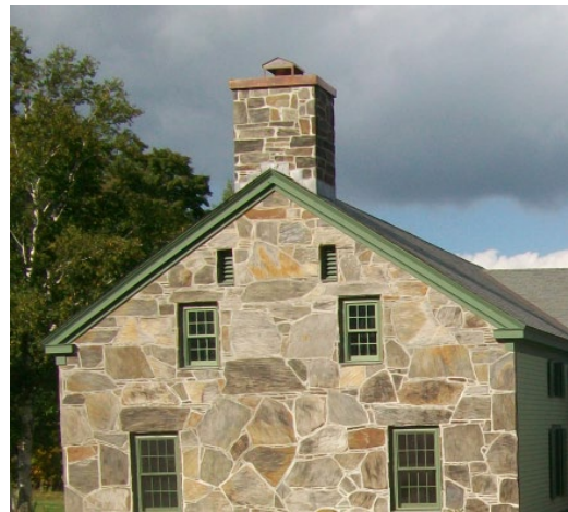
Gable end attic vents hold louvers. Courtesy of the Vermont State Historic Preservation Office.
