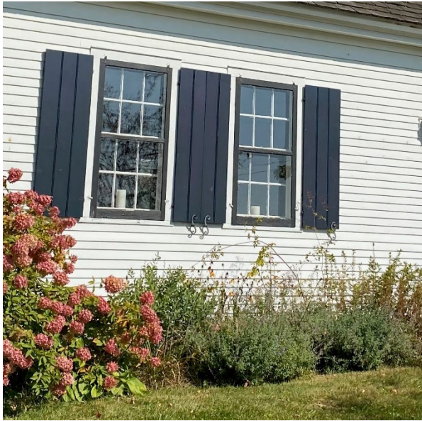
Operable wood shutters with shutter dog, framing removable storm windows. Courtesy of the Preservation Trust of Vermont.
