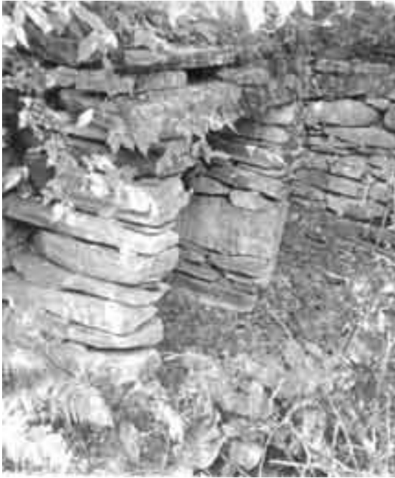
Left, Example of split arch chimney foundation—Chester; Right, Stone-lined well
